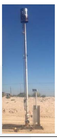
Aereon's Momentum Series, Unassisted Flare is used to burn off waste natural gas from a high-pressure separator. The technology used for this flare design allows for 100% smokeless combustion without requiring any utilities for operation. A highly reliable solar ignition package is utilized for convenience and dependability. A deflagration arrestor is also installed in the supply line to prevent flame backflash.
